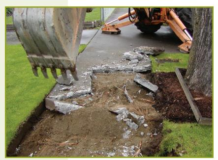
Sidewalk excavation due to tree root damage
