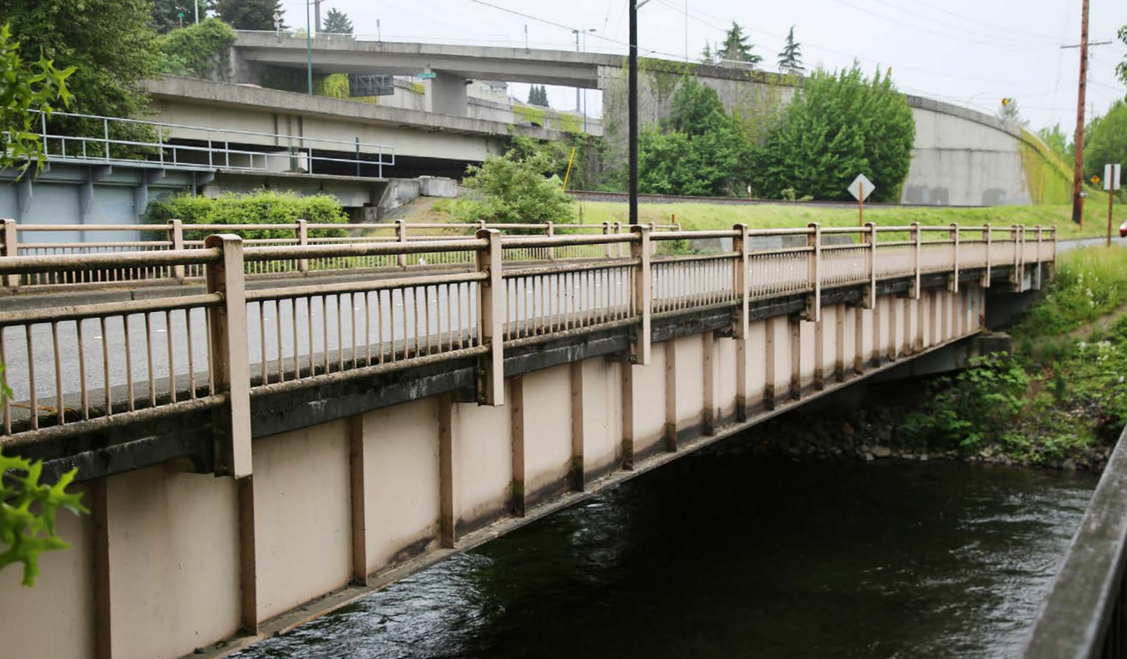
Houser Way Bridge
