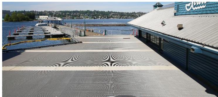
*The new north and south decks at Gene Coulon Memorial Beach Park are made of fiberglass and aluminium which allows sunlight to pass through, creating a more fish-friendly environment.*
