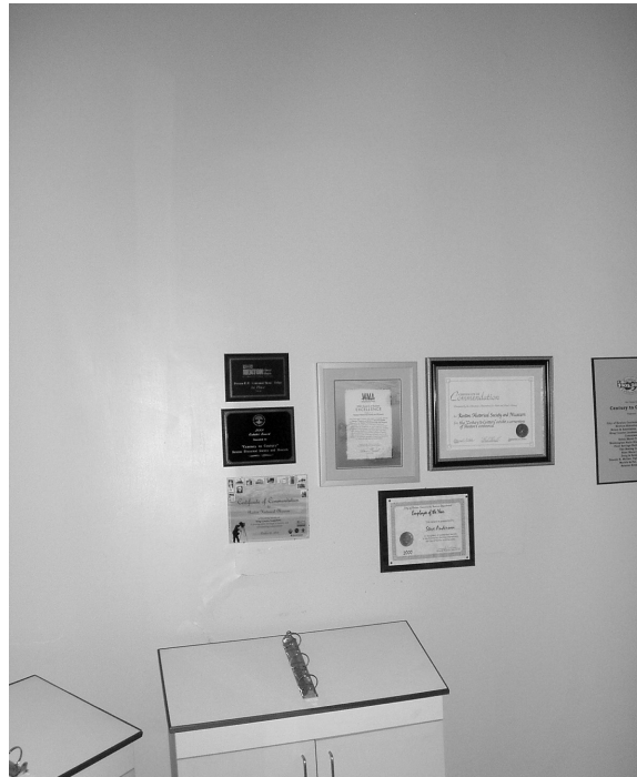
The “ghost” of the window corner is visible through the sheetrock – directly above table. Photo by author.
